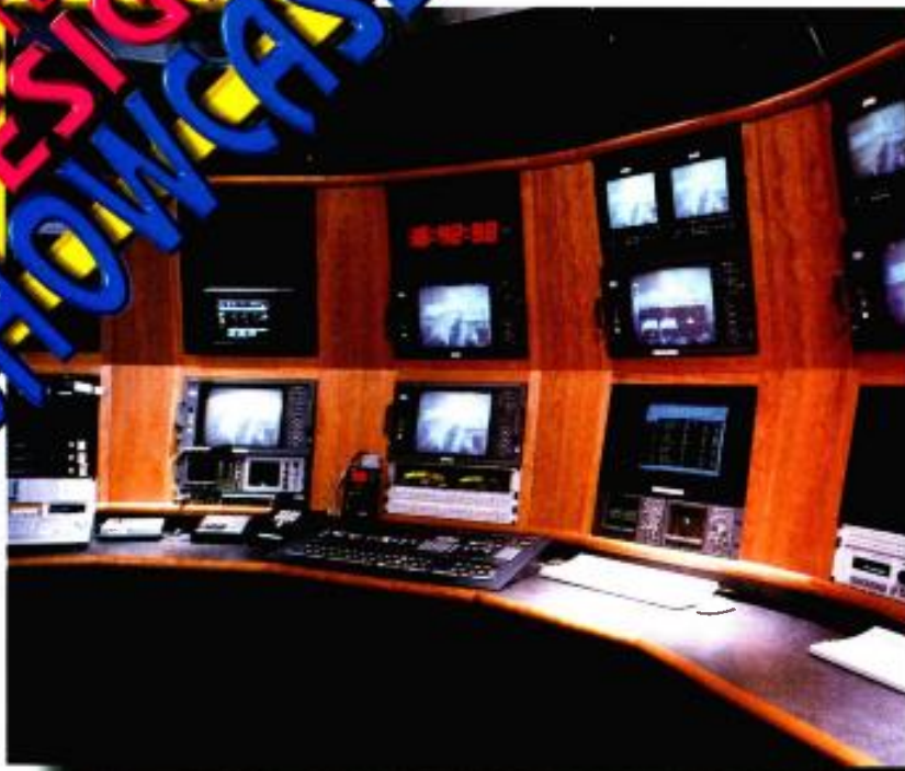
On-air switching is done with the BTS Philips Saturn digital switcher. This switcher provides a path to automated, multichannel operations.
